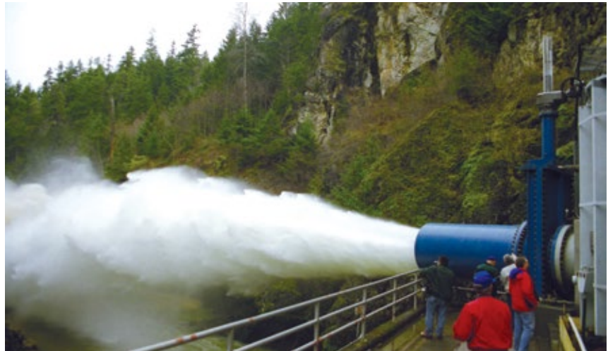
42" Jet Flow Gate, Head 800 Feet, La Grand Dam, Tacoma, WA
